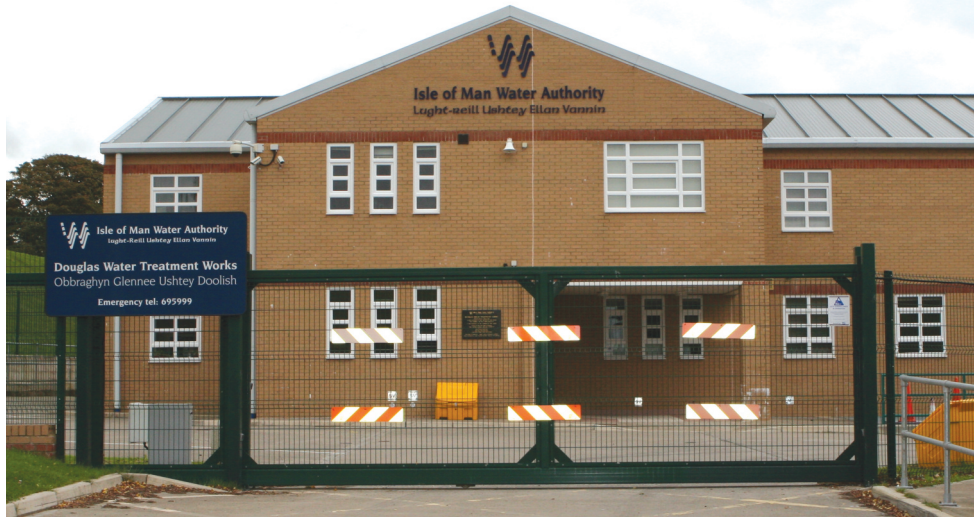
New water treatment plant in the heart of the constituency
